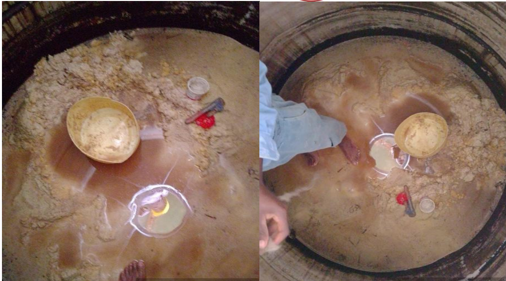
Pictures showing the cleaning and removing of the scalant at the Health Centre Water Tanks
