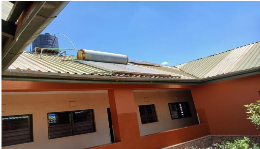
picture showing the Solar Water heating panel
