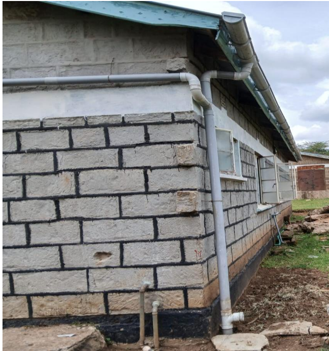
A picture showing the installed gutters
