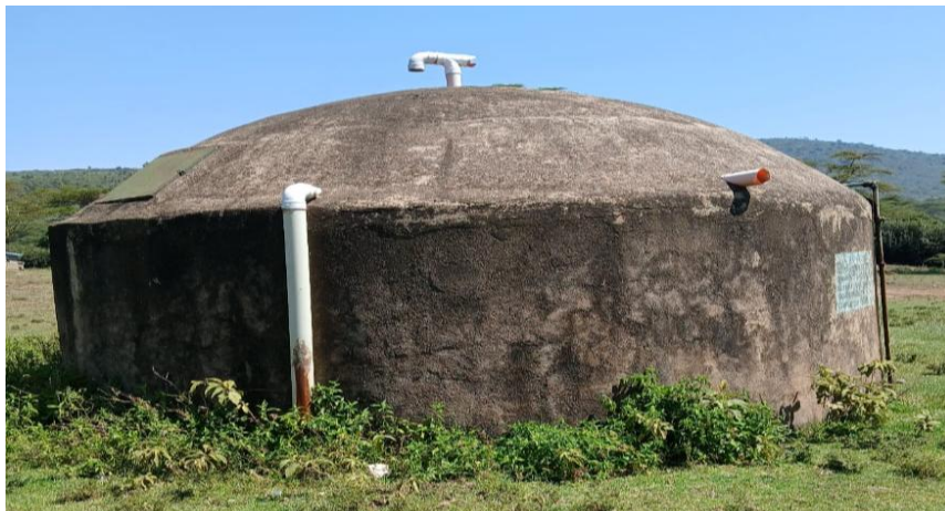
Picture showing the water holding Tank from the stream
