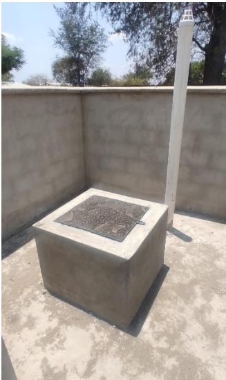
A newly constructed medical waste pit. Photo credit CRS staff
