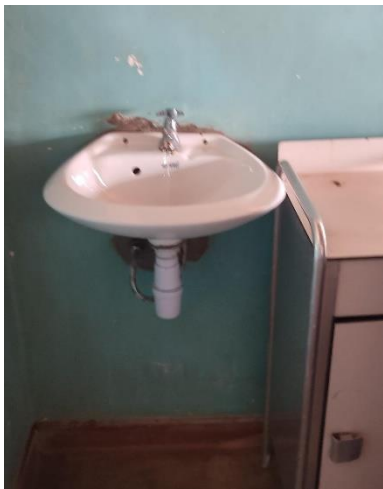
Sinks were installed in all wards. Photo credit CRS staff
