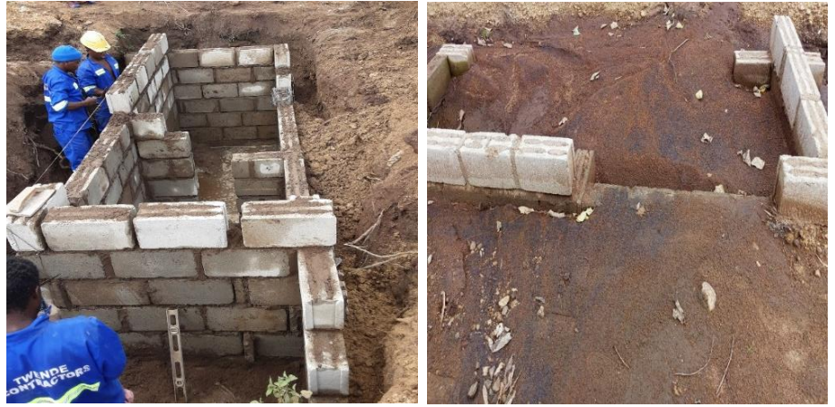
Latrine structure before the cyclone, left, and after, right. Photos by CRS staff
